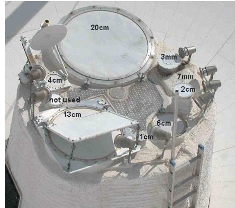
VLA instrument feed pedestal
