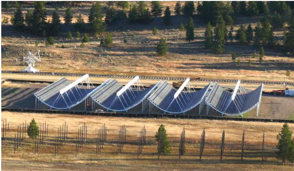
Figure 1: The CHIME telescope, currently nearing completion. Commissioning will begin in late 2016, and a dedicated FRB backend will be deployed beginning in early 2017. The multi-year CHIME-FRB survey will begin later that year.
