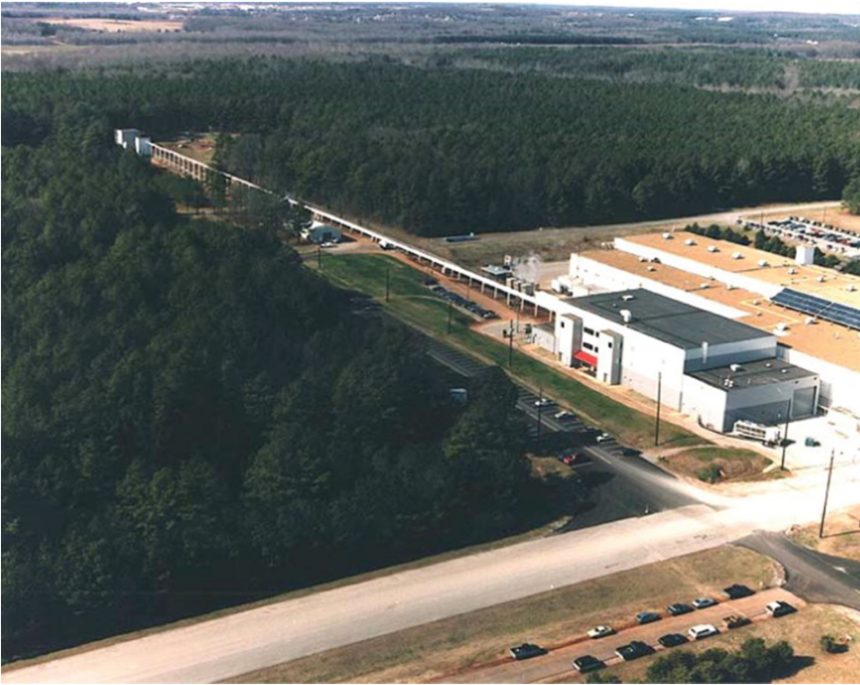
Figure 0.4. Aerial view for the X-ray Calibration facility used to calibrate the AXAF optics. The source chamber is toward the upper left, the 1700 ft-long pipe is in the center, and the building housing the vacuum chamber and the team working area is at the right. (Courtesy of NASA.)
